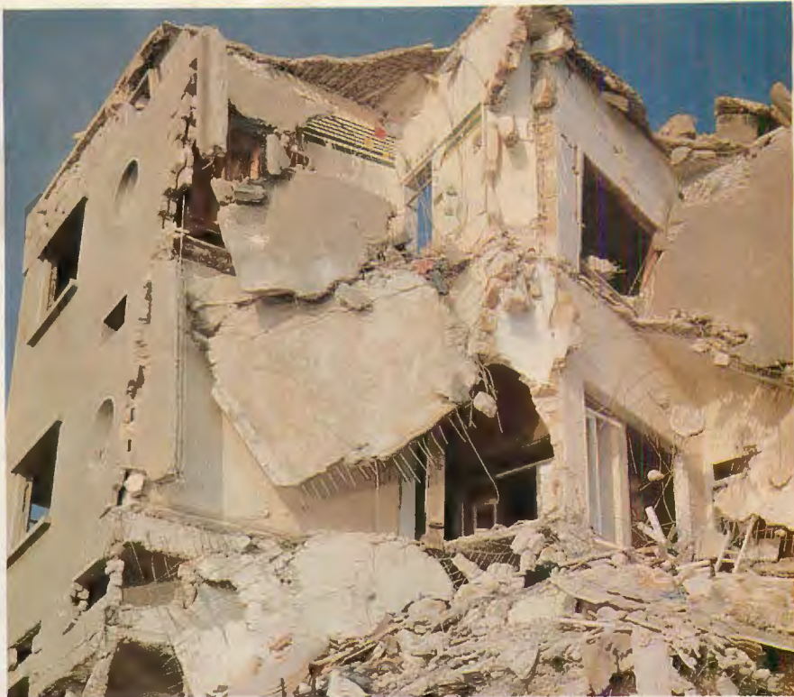
Beirut's broken buildings offer IDF snipers their best cover and their greatest danger. Photo: Jim Morris
